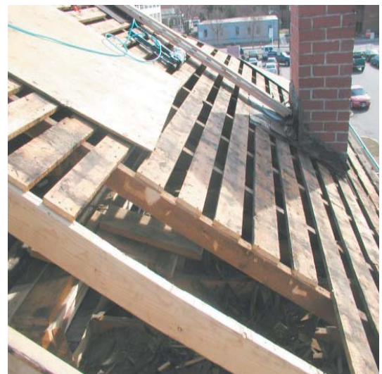
Urgent roof repairs performed once emergency building permits were issued
